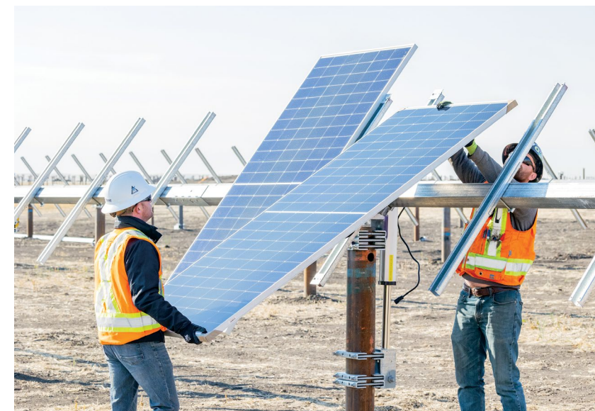
The first panels are installed at Michichi Solar in 2022, Drumheller, Alberta.
