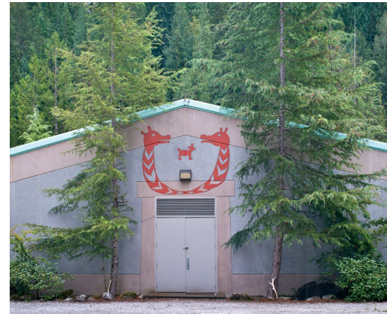
LEFT Celebrating the start of operations at Goulais Wind with partners Batchewana First Nation in 2015, Ontario. RIGHT The Sechelt Hydro longhouse-style powerhouse designed with partners shísháhl Nation, British Columbia.
