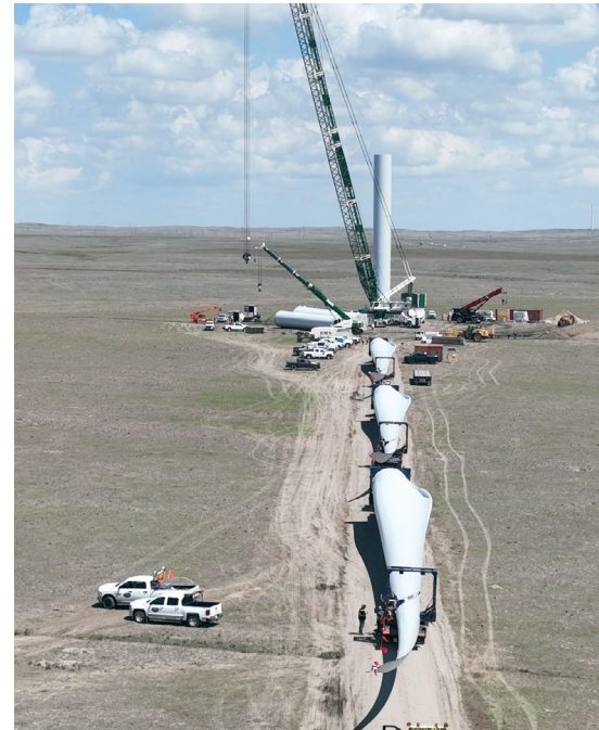
TOP LEFT Claresholm Solar. BOTTOM LEFT Kneehill Solar under construction. RIGHT A turbine going up at Buffalo Atlee Wind, Alberta.
