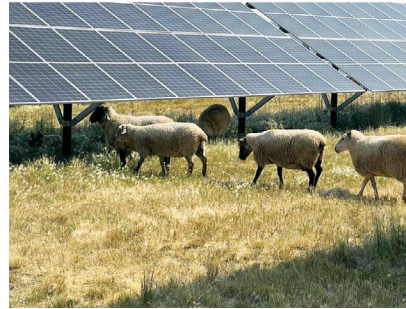
Sheep amongst the panels at Claresholm Solar.
